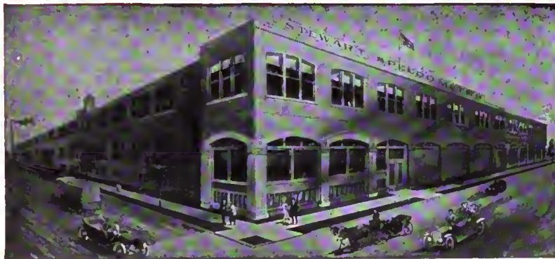
STEWART SPEEDOMETER PLANT SHOWING NEW ADDITIONS
